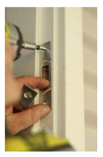
Close the door and using the key lock the door. If the lock hole has no restriction then it should lock effortlessly. Now go inside and repeat this process. This action should deadlock the internal snib, if it does not then there must be a restriction and it will have to be removed.
