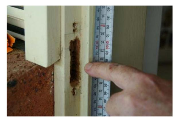
If you have an existing lock hole (1.6) from a previous door and you are confident that this has clearance from the existing lock, based on the Lock Above & Lock Below guidelines, then measure from bottom sill to the centre of the lock hole and deduct 4 mm. This will be the handle height. The centre of the lock tongue is the centre of the handle.
