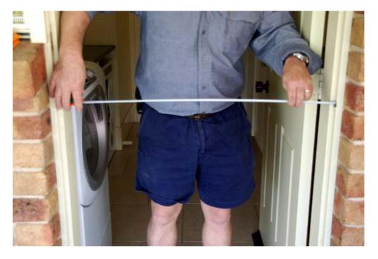
Hinge Bind: If your middle width is longer or shorter, creating a bow in or out at the middle, this must be corrected. For a bow in the centre the hinge can be packed out (0.5 mm Hinge Packers are available). For a bow out, the hinge will have to be let in, this must be done by altering the timber door frame, however you can request to have the middle hinge raised, lowered or supplied with the door and not affixed.
