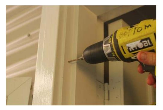
Hold the door in place. Using a cordless gun, screw through hinge centre elongated hole into pilot hole and screw up tight (1.3). Repeat the same process using the centre hole of the bottom hinge. Now close the door onto the jamb and stand outside. Adjustments up and down can be made now if necessary by loosening the two screws. Once you are happy with the doors position then pilot drill and fix all remaining screws to the hinges.
